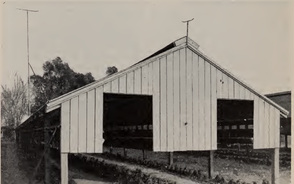
Fig. 41. Four-row, single-tier cage hen house. Note automatic drip valve watering system which works well for birds in cages or on wire floors. Note also the sprinklers on roof.
